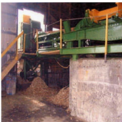
Post and chains – unacceptable
